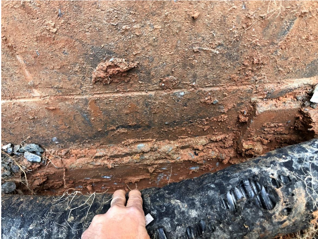
Block resting on concrete wall stepping down
