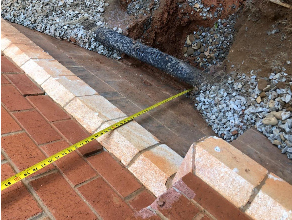
Area where backfill partially removed. Measuring down to top edge of concrete wall.
