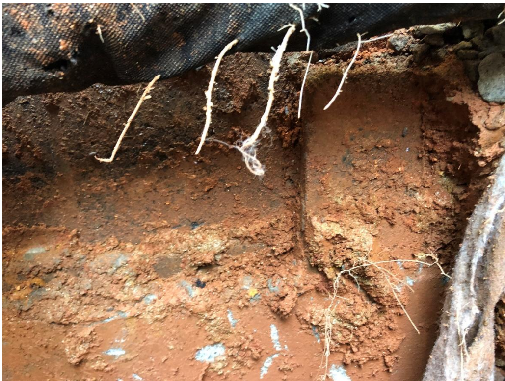
Block resting on concrete wall stepping down
